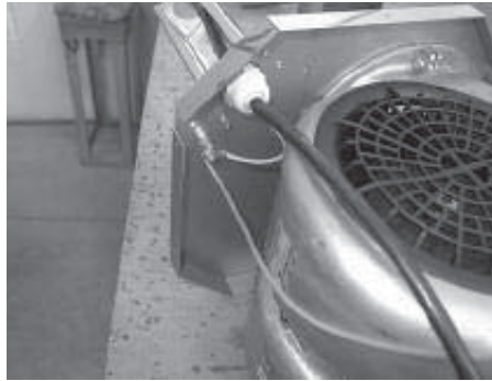
7. Attach grounding wires from junction box and motor to grounding screw as shown.
